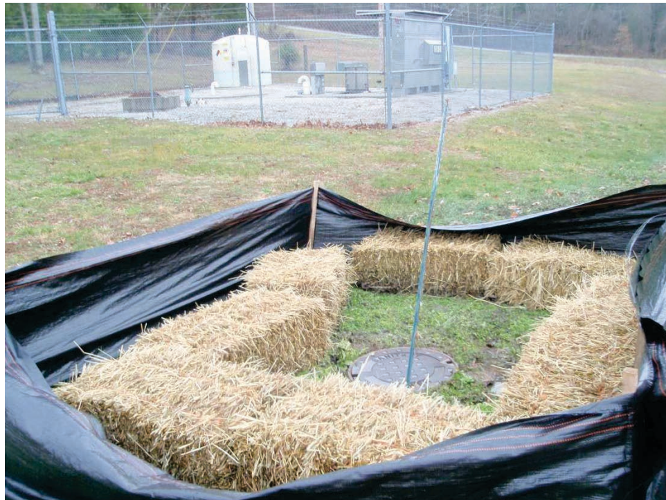
Figure 8. Southwest Pump Station Overflow Point
