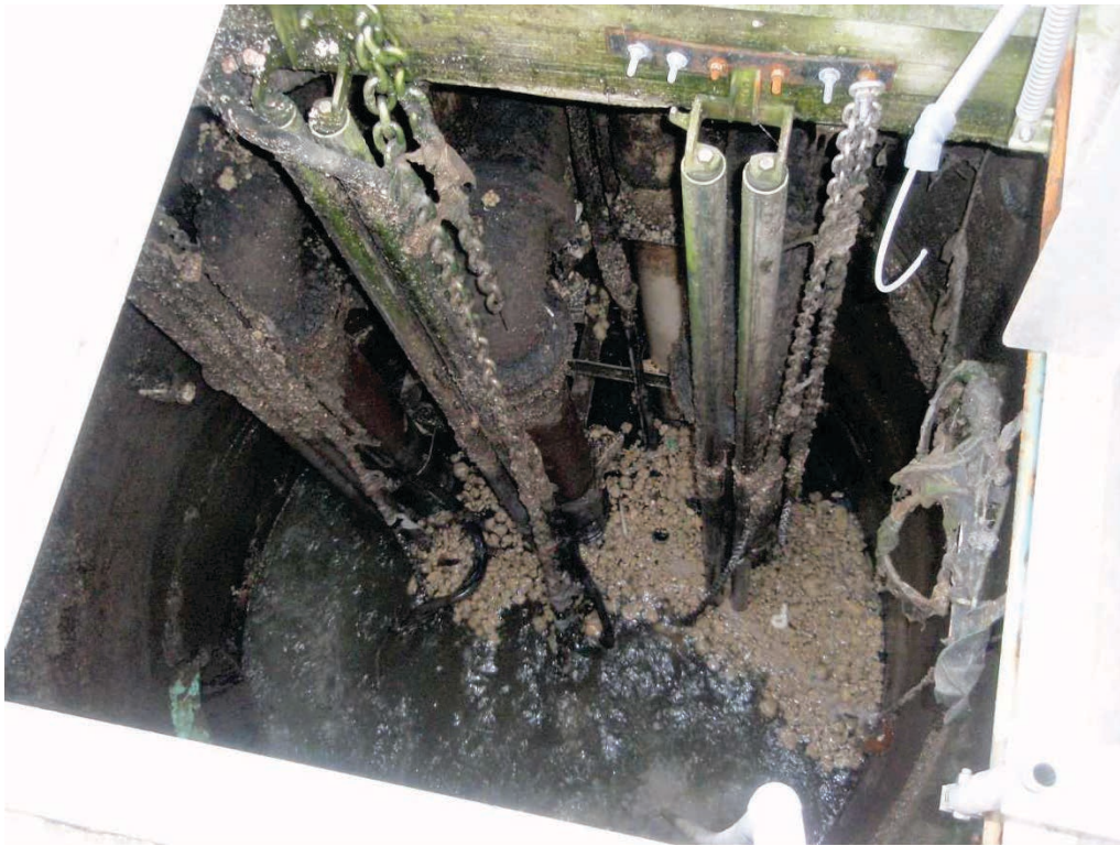
Figure 10. Southwest Pump Station Wet Well
