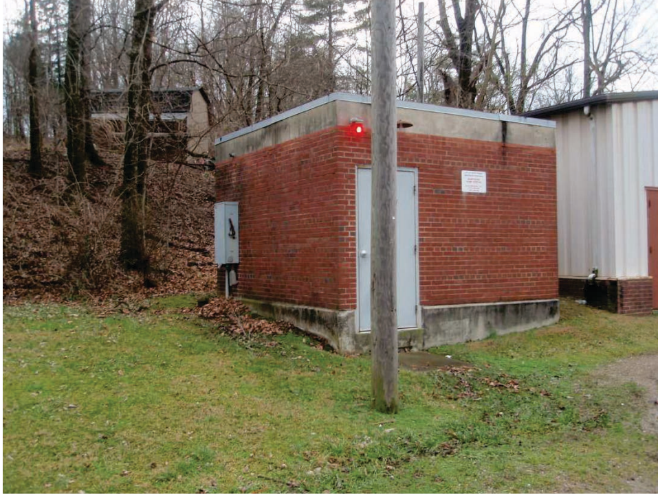
Figure 3. Northeast Pump Station
