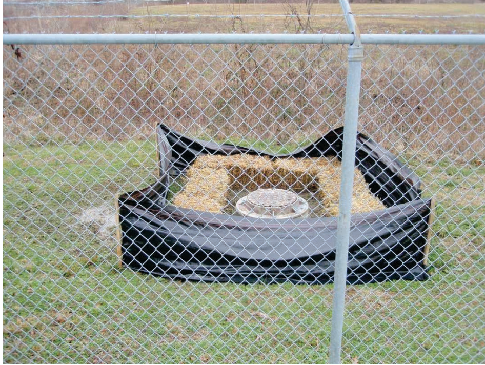
Figure 5. Northwest Pump Station Overflow Point
