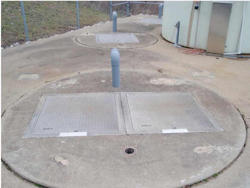
Figure 4. Northwest Pump Station Wet Well
